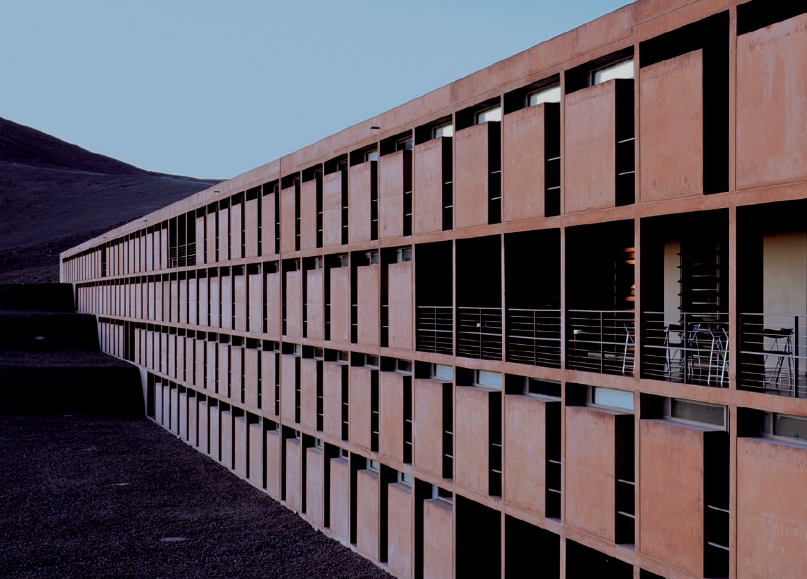
ESO Hotel, Cerro Paranal, Chile. Pigment: 2 % Bayferrox® 600 N, applied to cement. Concrete: compression strength class C20/25 (B25) and C27/37 (B35).
